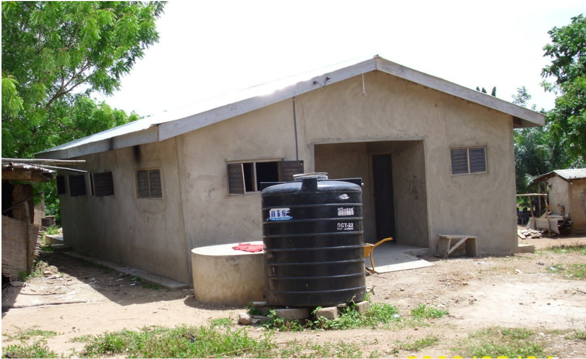
Construction of 10-Seater WC toilet at Todome
