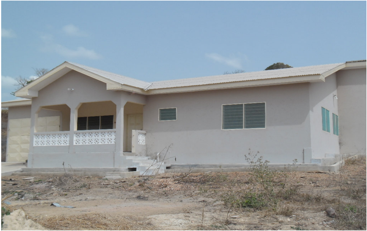
Construction of Senior Staff Bungalow No.2 at Tsyokpokope, Kpeve
