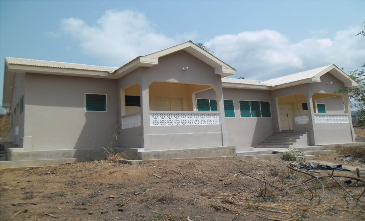
Semi-Detached Staff Bungalow No.2 at Tsyokpokope, Kpeve
