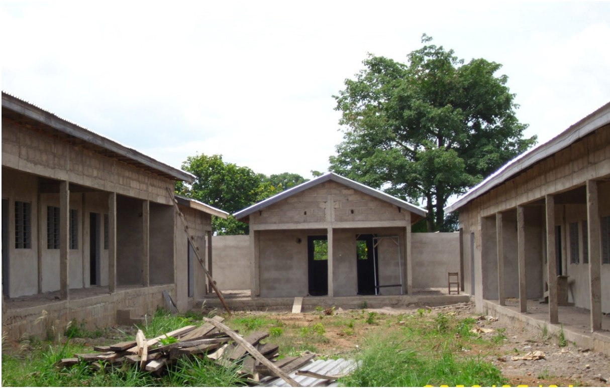
Construction of 8-Rooms Boys Dormitory at Peki SHS
