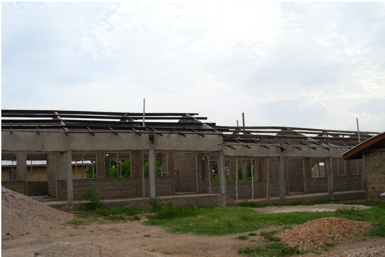
Construction of 6-unit classroom block at Dzemeni E.P. 'B' Primary School
