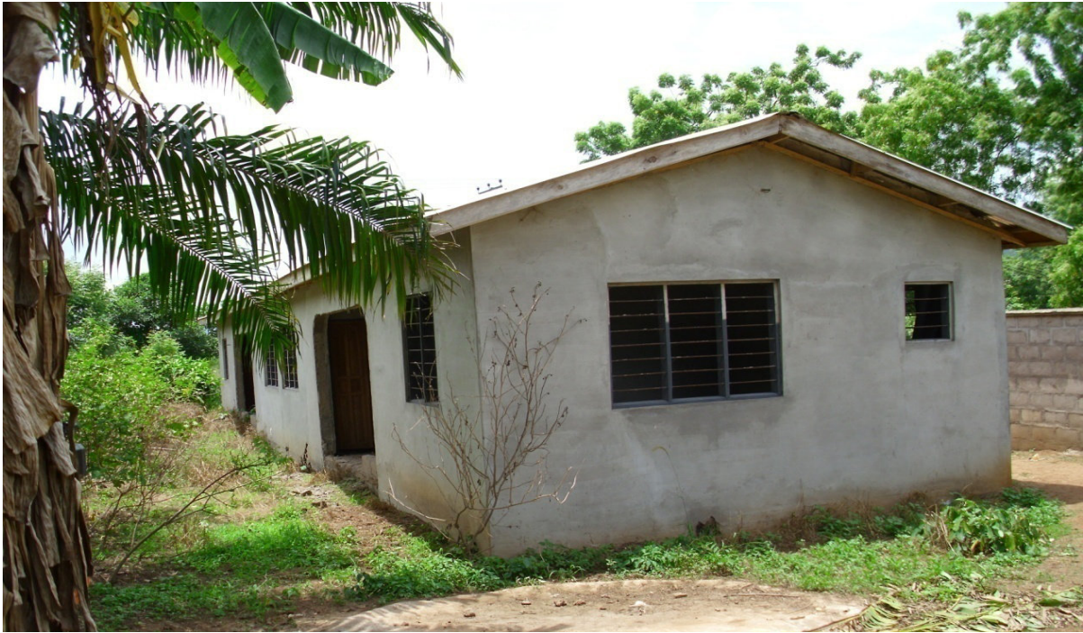
Construction of 2-unit Nurses Quarters at Peki Government Hospital
