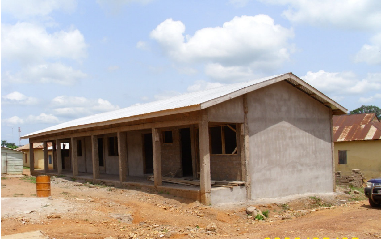
Construction of Kindergarten block at Peki-Wudome Primary School
