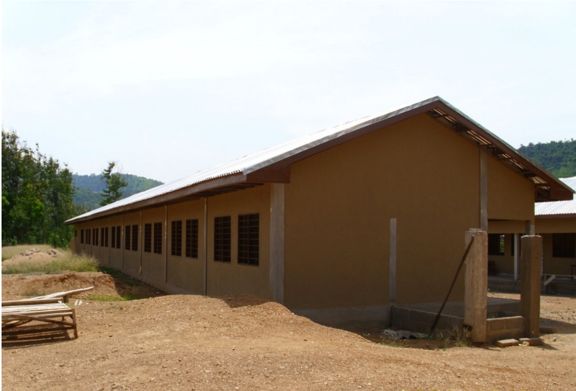
Construction of 8-Rooms Girls Dormitory with ancillary facilities at Kpeve SHS
