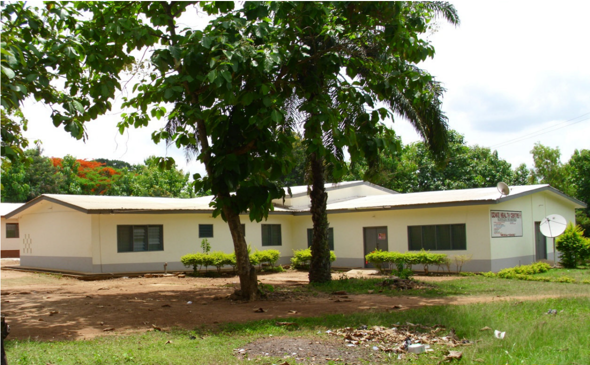
Renovated Health Center at Peki-Dzake
