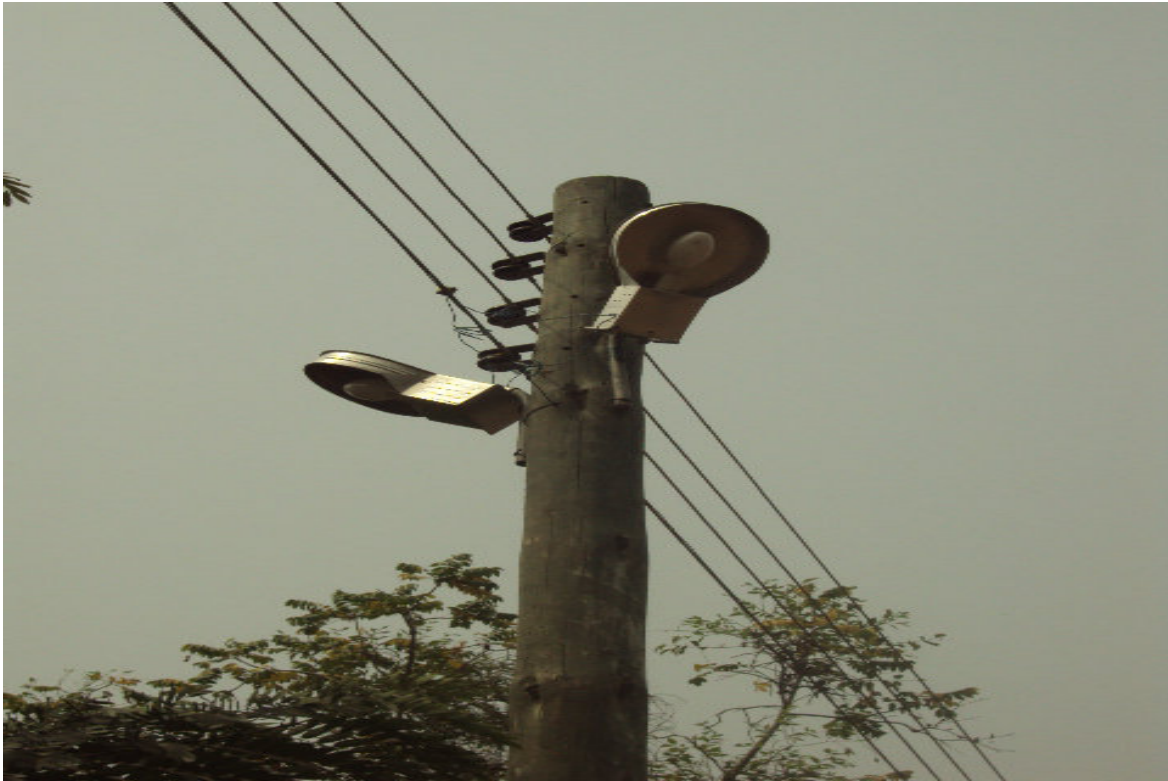
Installation of Street Lights at Sanga, Tsiyinu, Peki-Dzake, Kpeve, Dzemeni & Others
