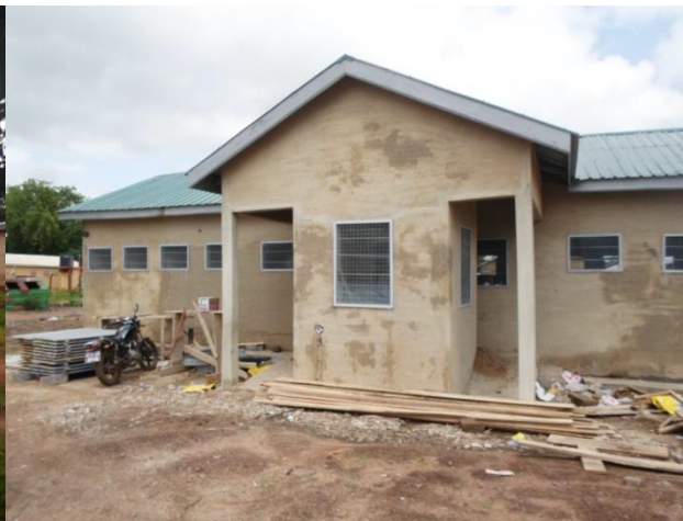
Ultramodern toilet at Tumu lorry station-DDF
