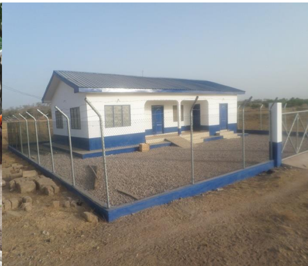
Office of Wellembele small town water system
