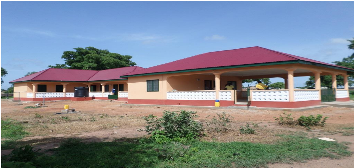
CHPs at Dimajan under DACF
