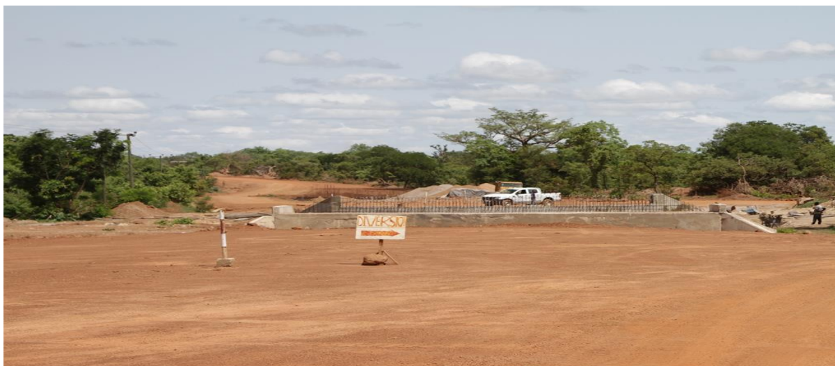
Tumu –Navrongo road under construction
