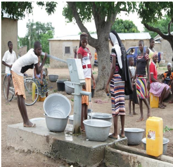
Installed Borehole at Sentie
