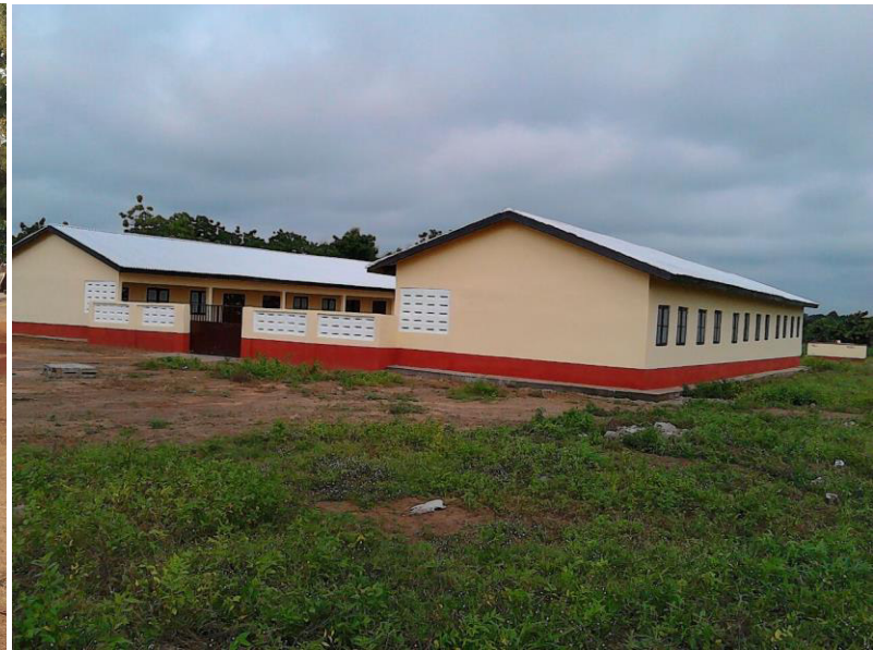
6-Unit Classroom @ Nansoni
