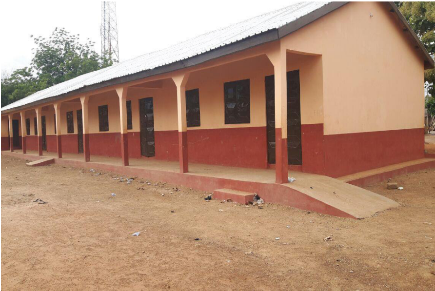
4-Unit Classroom with store and office @ Chereponi
