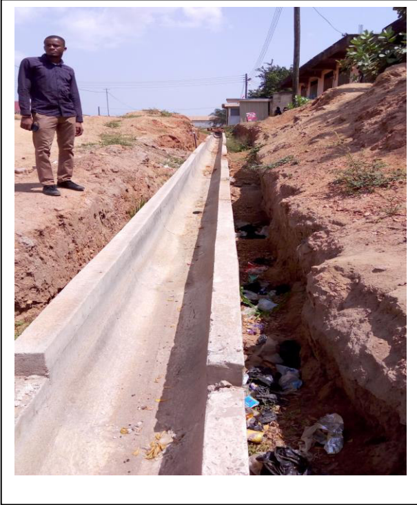
5. Construction of drains, Comm. 12
