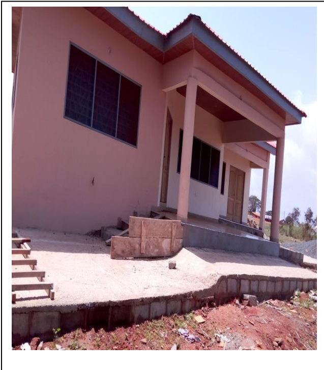
1. CHPS Compound at Bankuman
