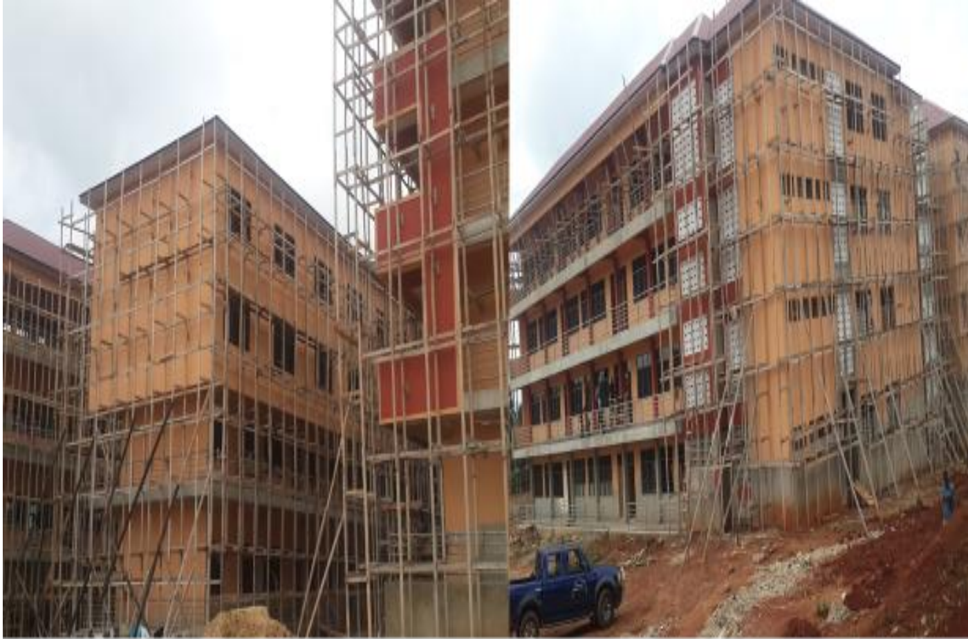
CONSTRUCTION OF FODUA COMMUNITY SHS
