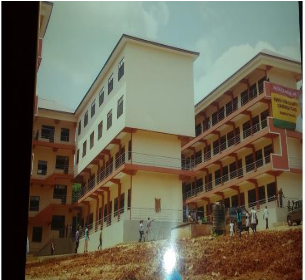
COMPLETED FODUA COMMUNITY SHS
