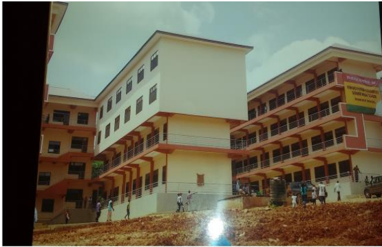
COMPLETED FODUA COMMUNITY SHS
